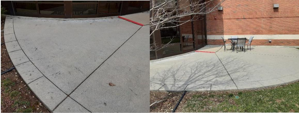
2. **Curb Repair** – Approximately 20' of concrete curb damage requiring replacement. Expected solution is removal and remolding of selected areas.
